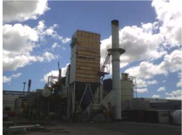
Forest Enterprises Australia (FEA) sawmill at Bell Bay
