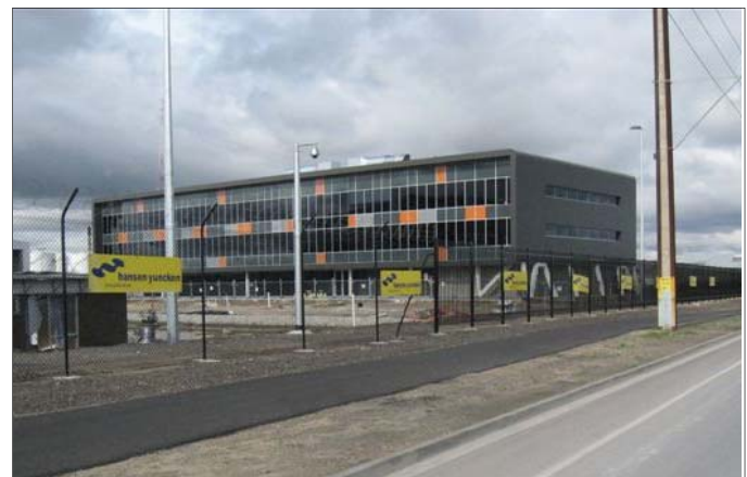
The new submarine base facility in Port Adelaide built by CFMEU FFPD glaziers
